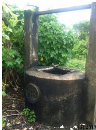
An unprotected concrete bucket well funded by the World Bank in the 2000s
