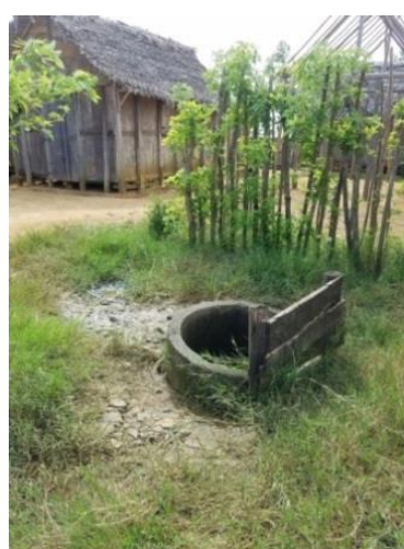
One of the two open concrete wells in Ambodivoara
